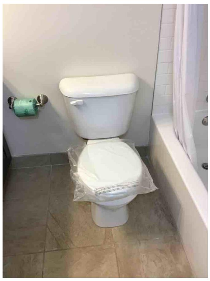
Use dye to check leak, adjust or change flapper, Fluid Master Supply Lines/Replace Plastic Lines
