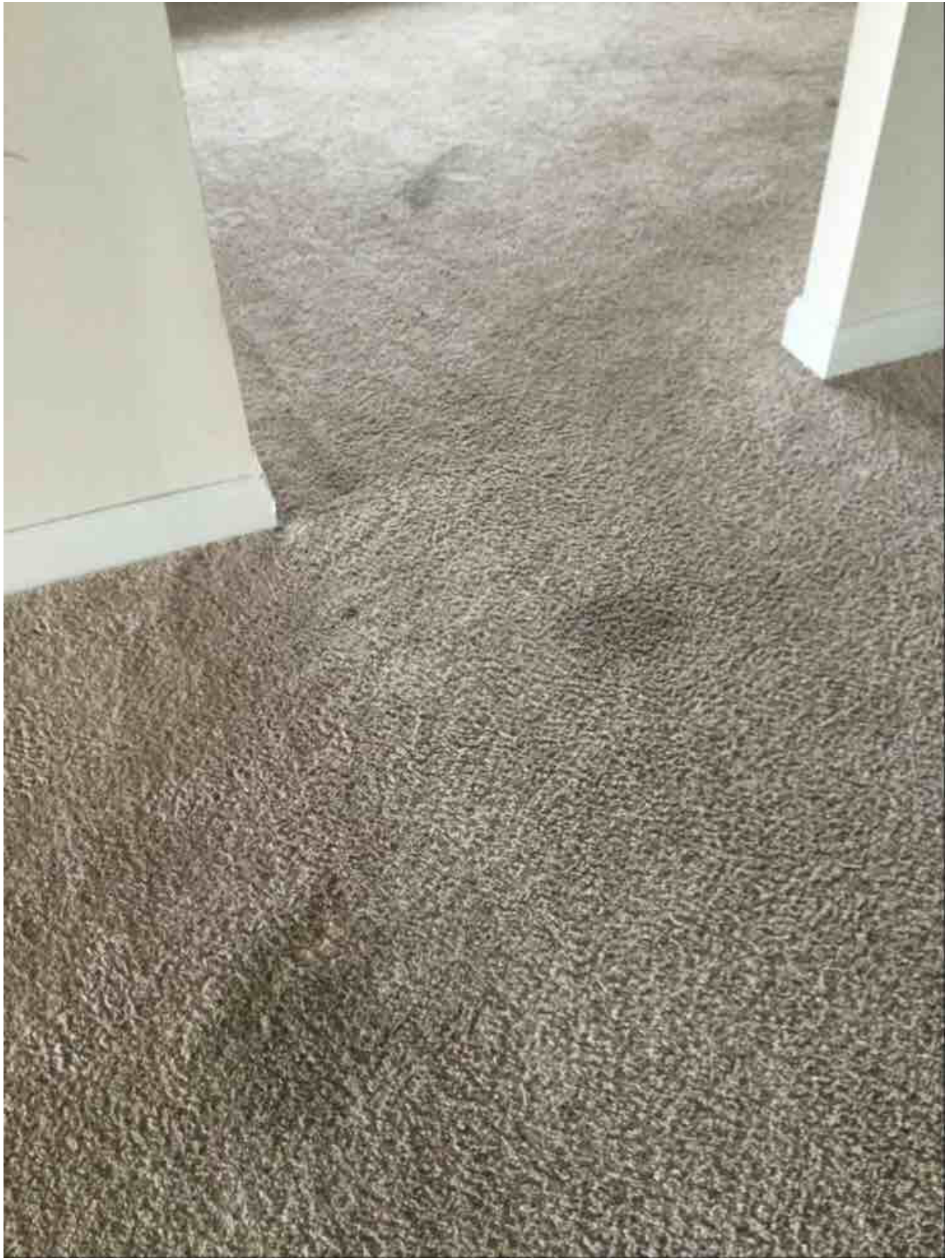
Stain Removal: Not Ok
