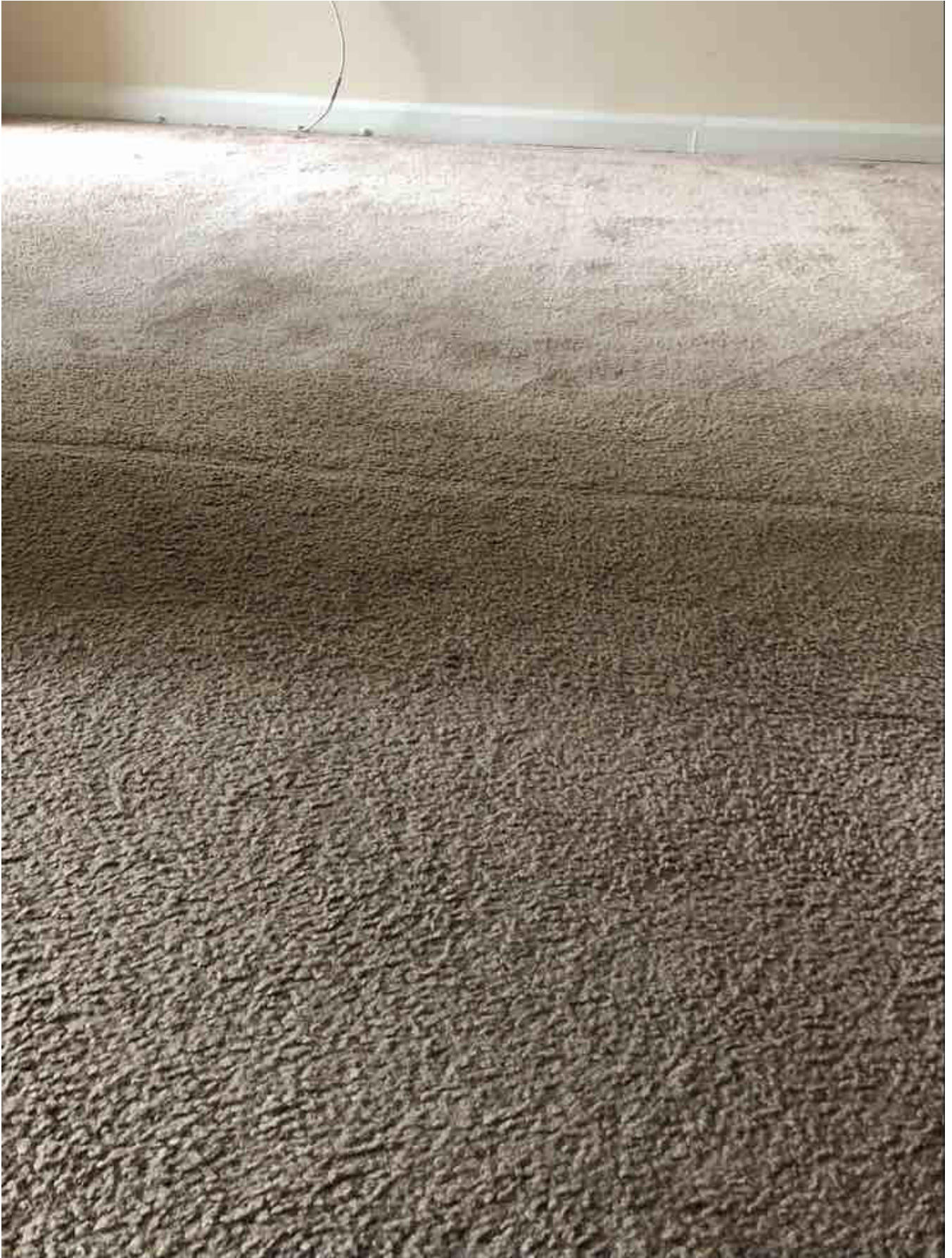
Stain Removal: Not Ok
