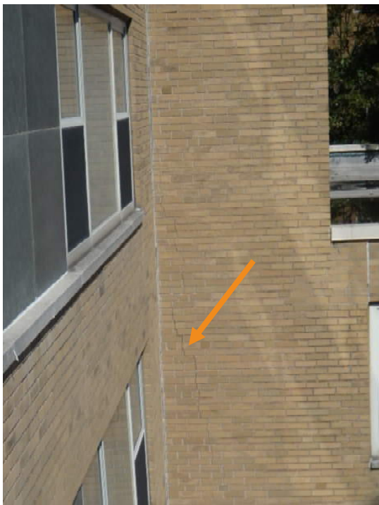
Photograph 16. Crack in brick veneer on the south facing side of the center stair tower on the east facade
