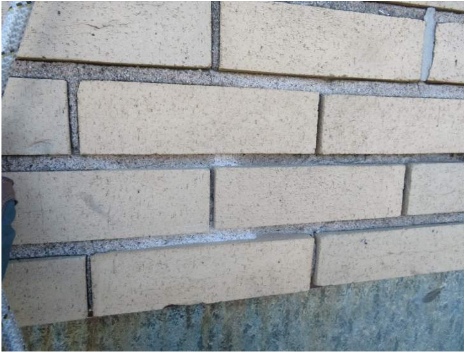
Photograph 23. Eroded mortar joint between brick units
