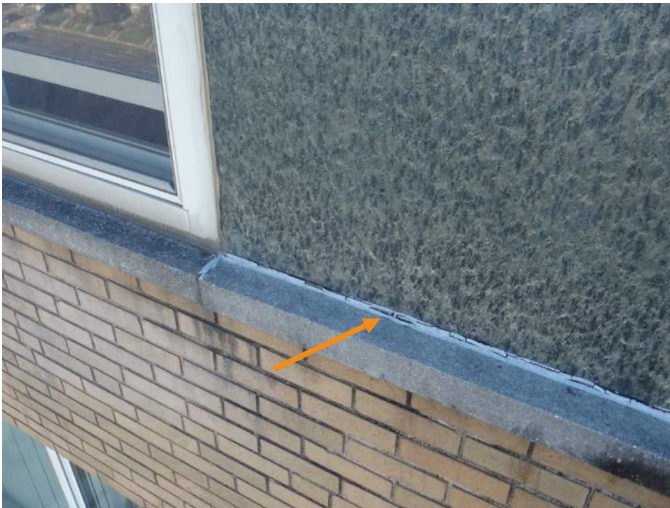
Photograph 28. Adhesive sealant failure between greenstone panel and precast stone sill
