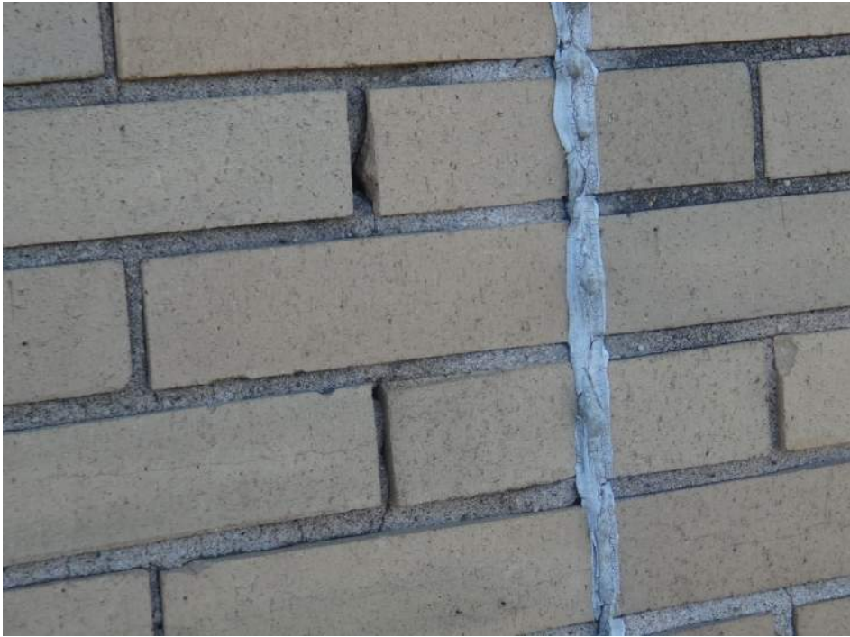
Photograph 25. Deteriorated sealant at control joint
