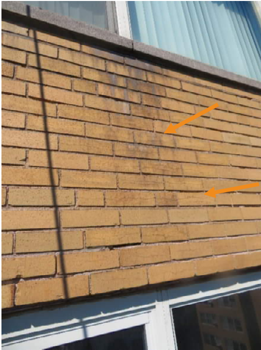
Photograph 15. Cracked and scaled brick on east facade below open windowsill joint
