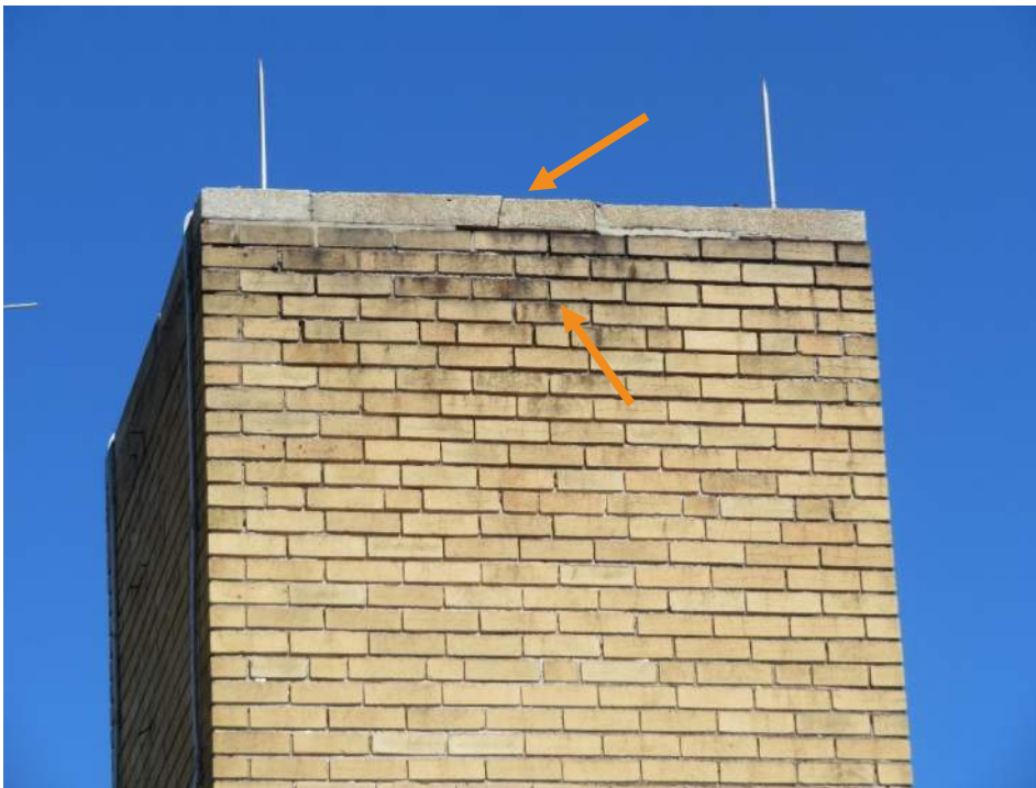
Photograph 14. Cracked coping stone units and brick bulging at the top of the chimney
