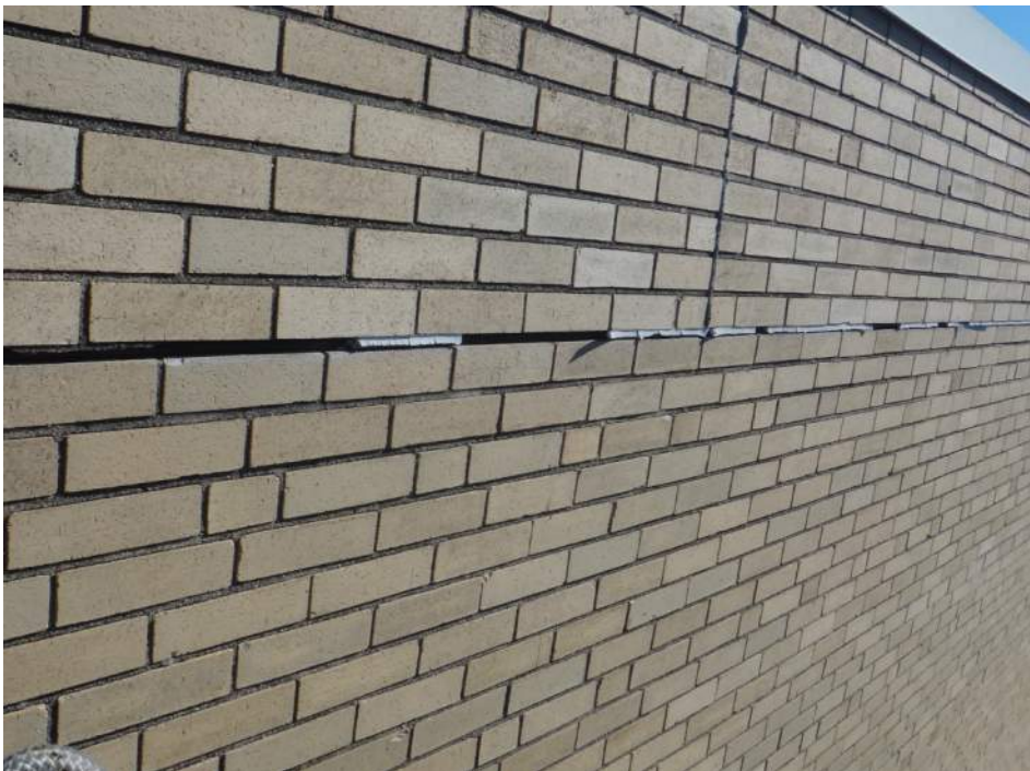
Photograph 12. Deteriorated sealant along the length of the steel relief angle
