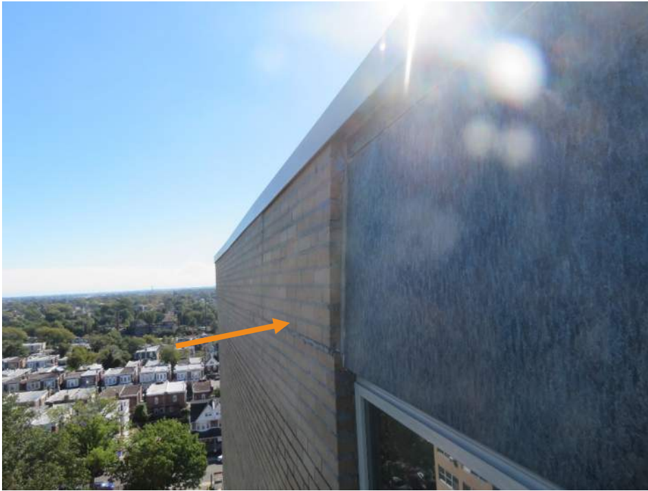
Photograph 11. Parapet wall leaning back on the north facade
