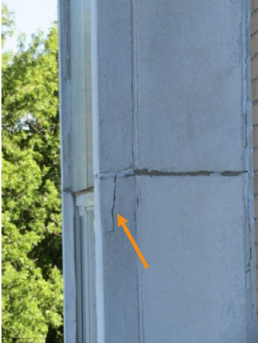
Photograph 19. Incipient spall at cast stone at west facade
