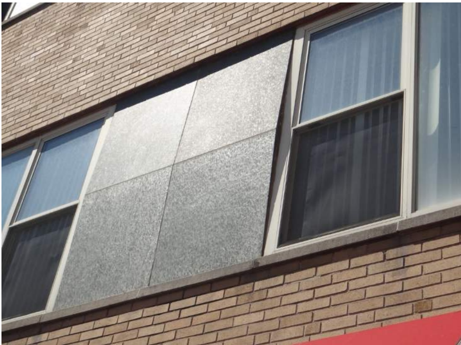
Photograph 6. Greenstone panels bulging along the horizontal joint
