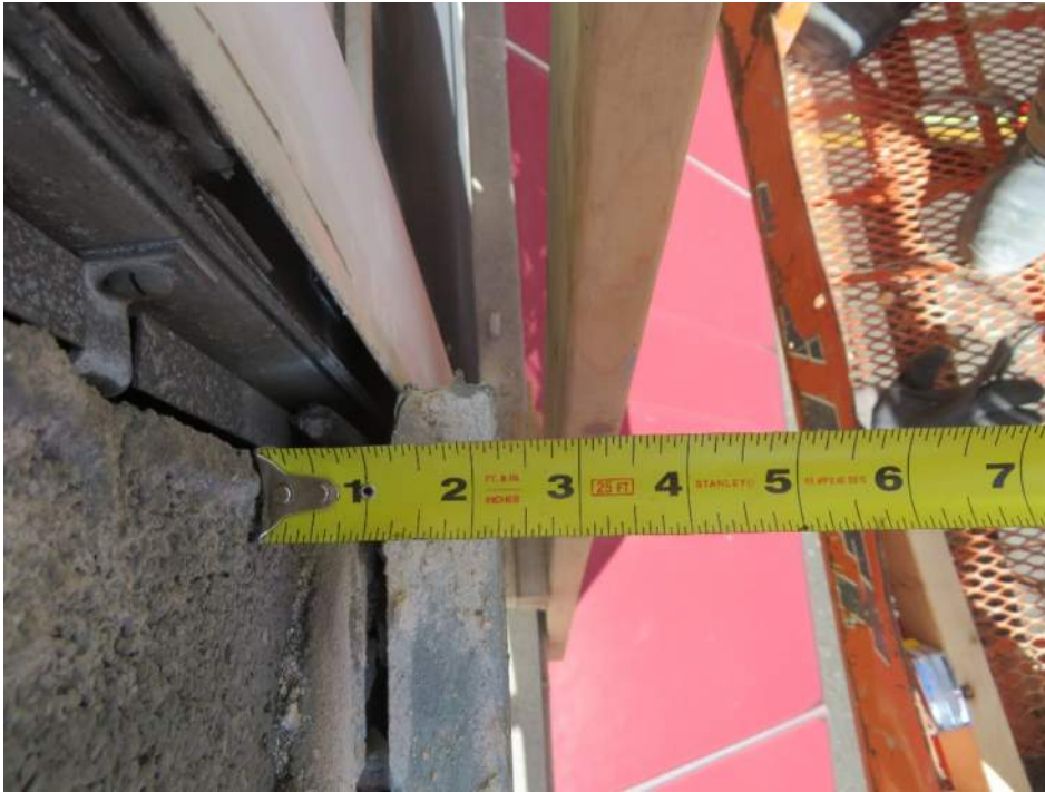
Photograph 7. Photograph of the CMU backup wall measurement where it was bowed at the center of its height
