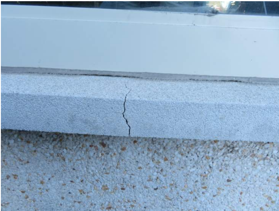
Photograph 18. Crack in precast stone sill on the west facade
