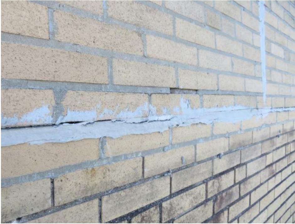
Photograph 27. Adhesive sealant failure along relief angle
