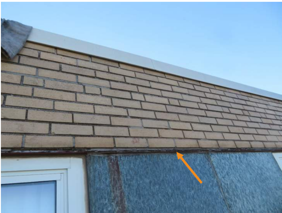
Photograph 10. Corroded steel lintel above twelfth-story windows
