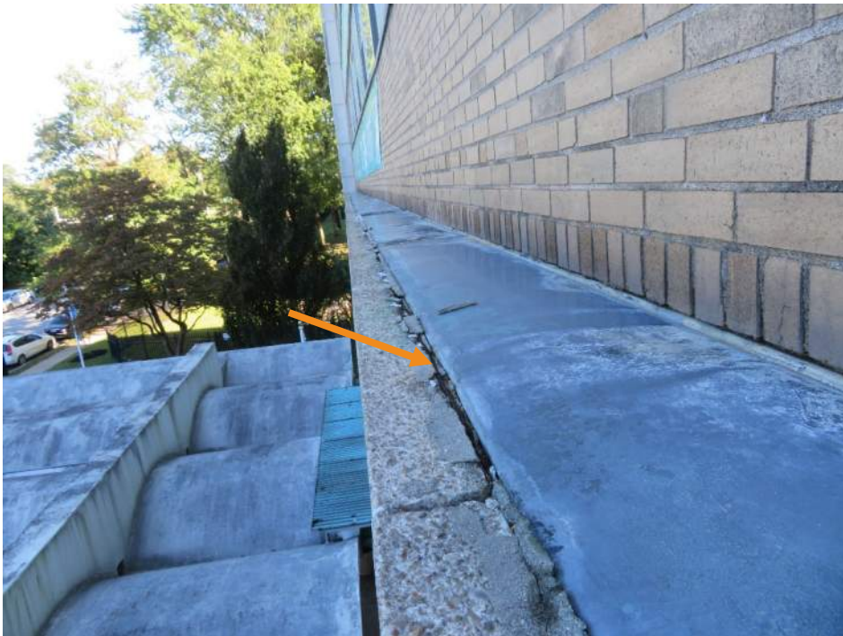
Photograph 24. Deteriorated mortar joint along top edge of precast surround on the west facade
