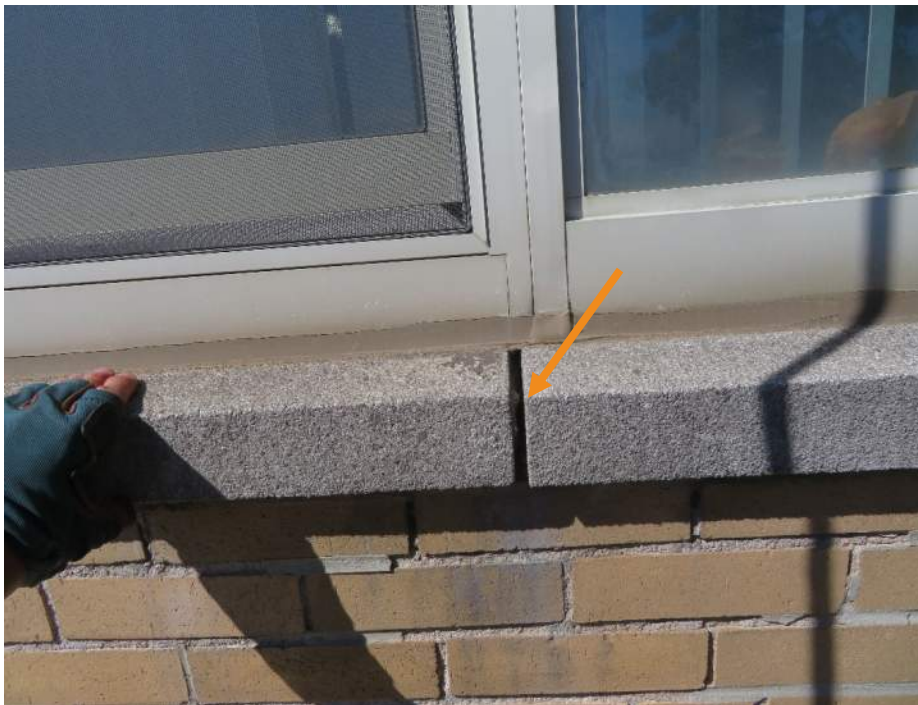
Photograph 22. Voids within joints between precast stone sill units
