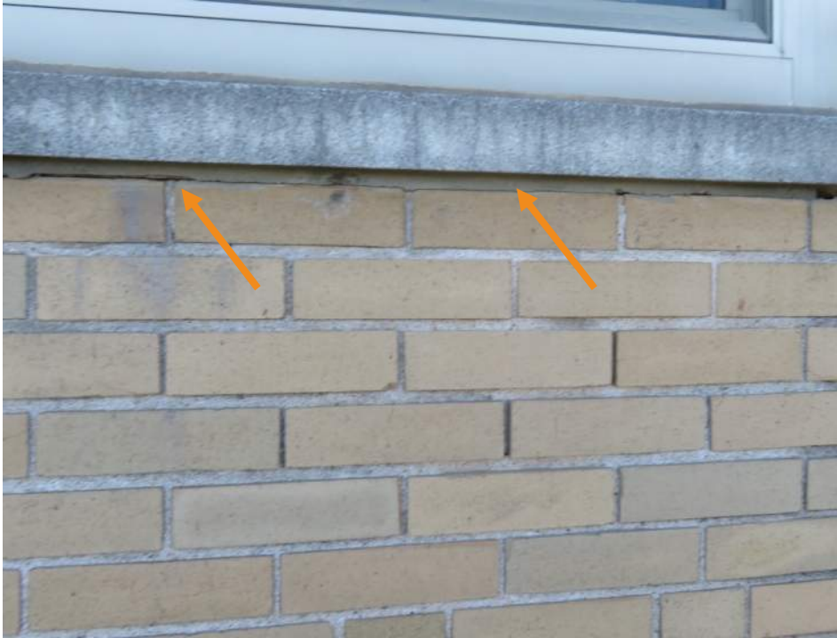
Photograph 29. Sealant present below precast stone sill
