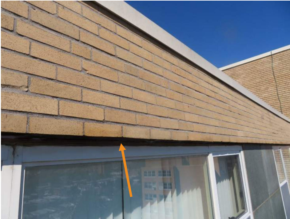
Photograph 9. Severely corroded steel relief angle
