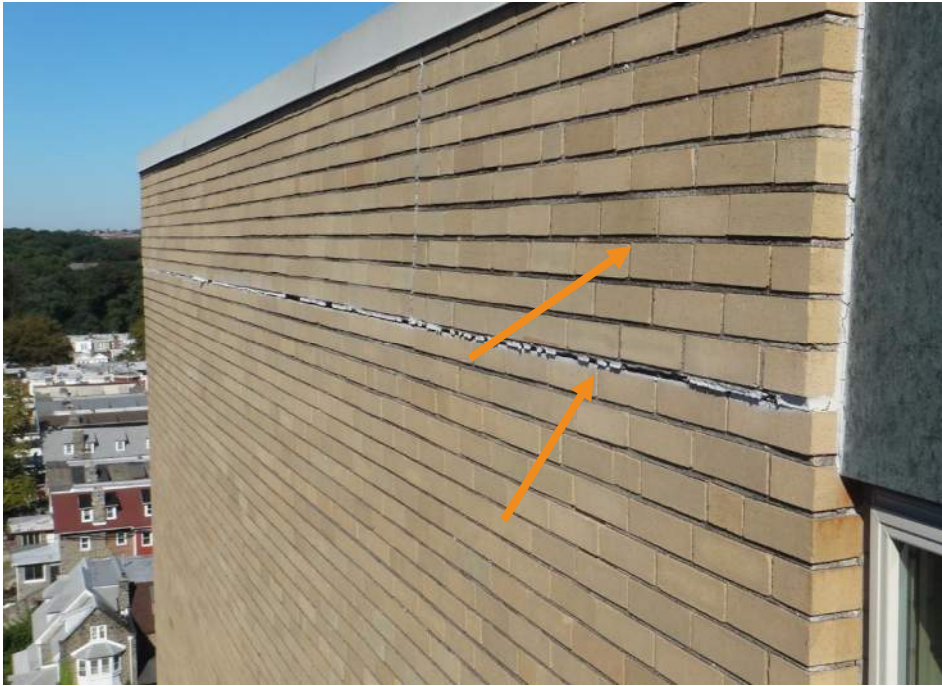
Photograph 13. Displaced/bulging brick parapet wall above relief angle on the south facade and sealant installed along toe of angle
