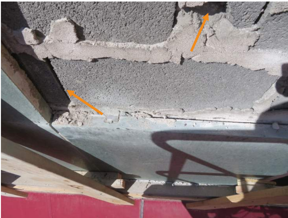
Photograph 30. Voids in CMU back-up wall
