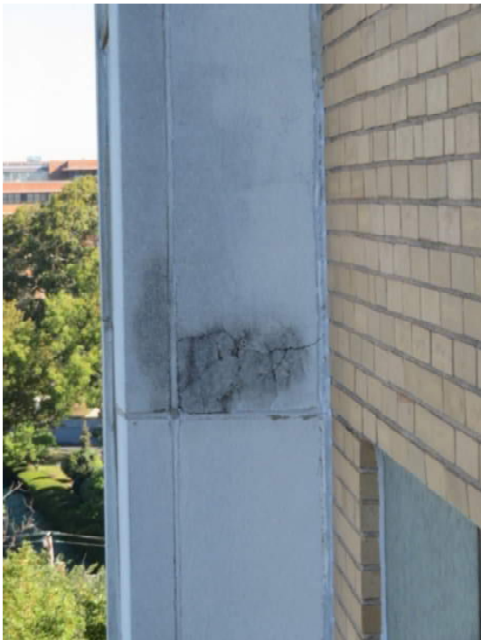
Photograph 20. Crack in cast stone on west facade
