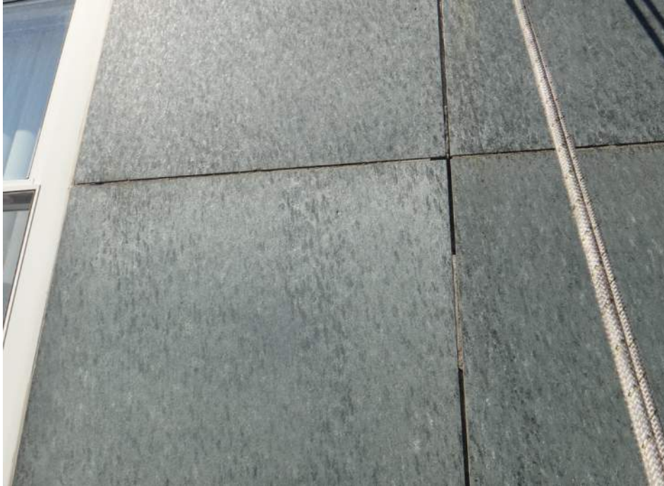
Photograph 21. Deteriorated/open mortar joints between greenstone panels
