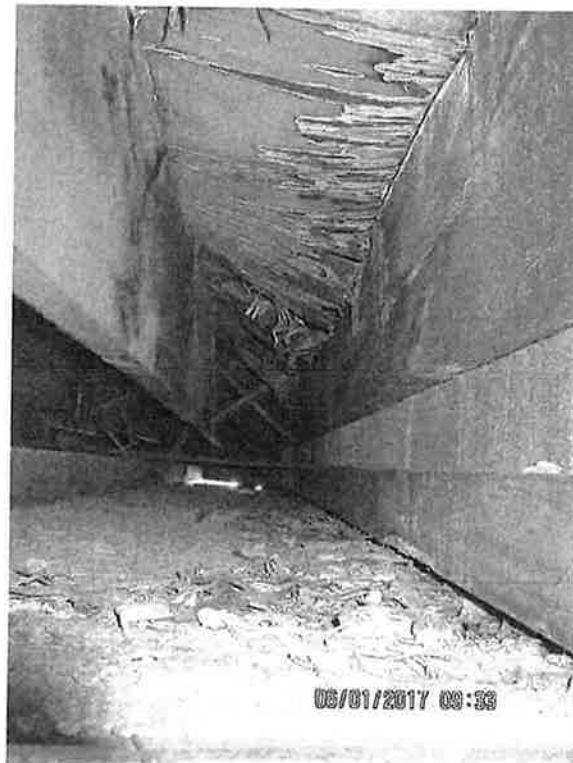
Typical roof level water damage
