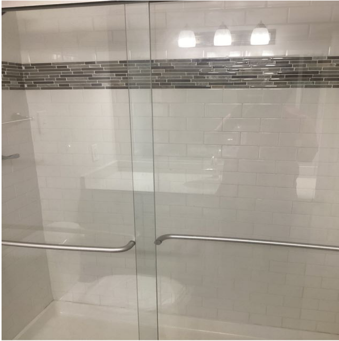
Amenity Name: Bathroom Upgrade
